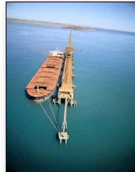
❖ *Deepwater port design optimised to accommodate “China-max” bulk carriers*
