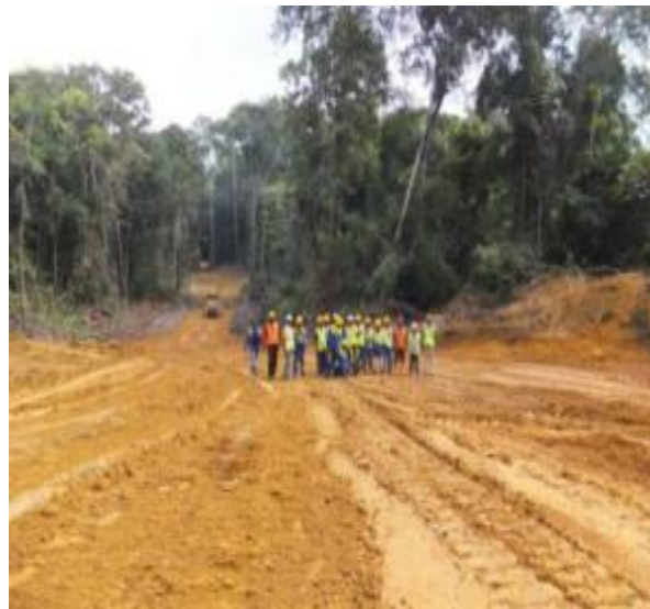
Construction of access road leading to the Lolabe Port
