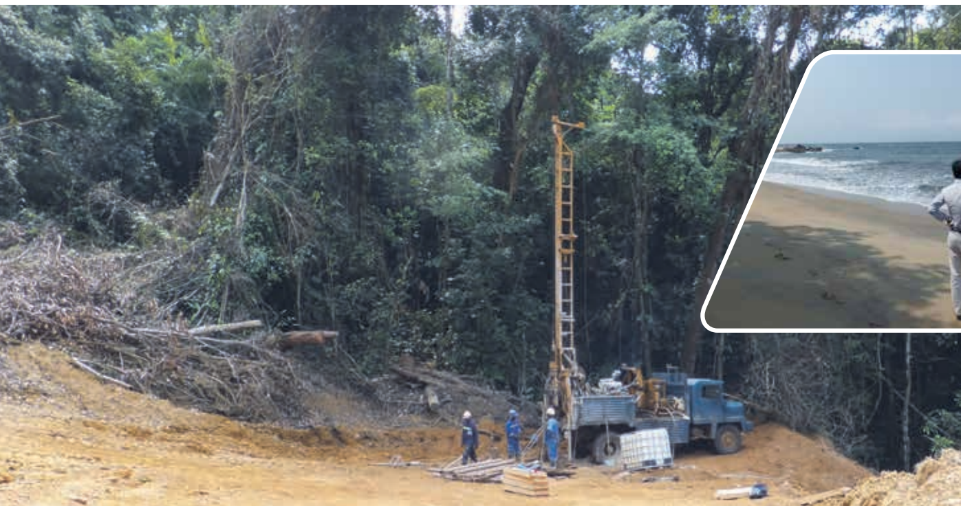
Geotechnical drilling and site inspection at Lolabe.
